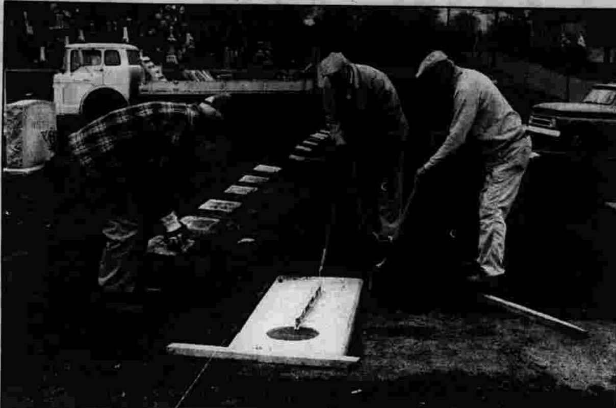
HEAVY STONE — Crewmembers from the Manchester Monument Company prepare the foundation for a memorial stone in East Cemetery. From left to right, George Adams, "Barney," and Stanley Murawski.
